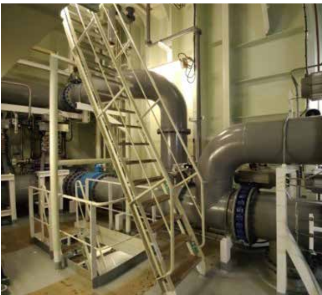
Images above: West Vela on-site installation.
