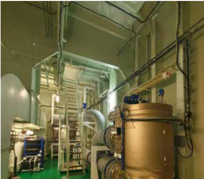
Images above: West Auriga on-site installation.
