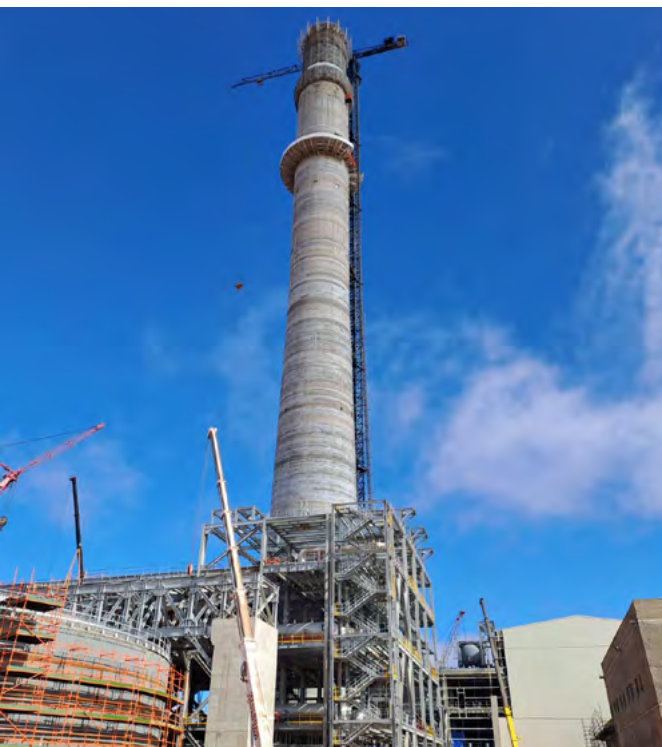
Images above: Construction of SEPCOIII Redstone CSP plant
