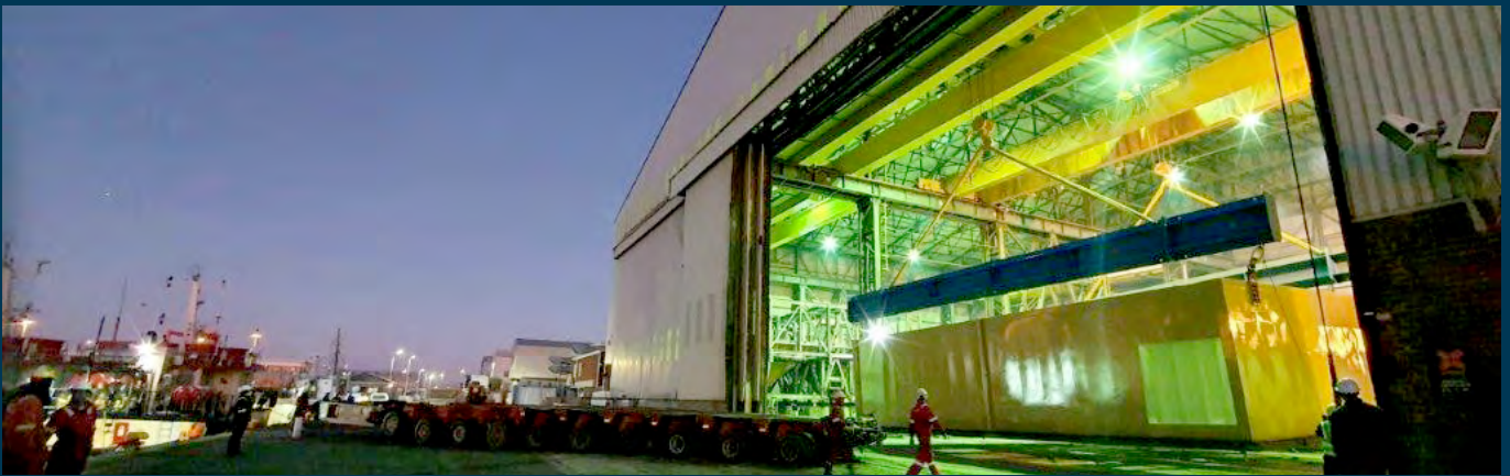
Cinco Engineering Workshop located at Cape Town Harbour, South Africa
