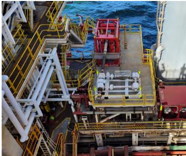
In total 13 scopes were awarded to 3C Metal. The main scopes included the rig mud gas separator (MGS) U-tube piping, integration of a second MGS with buffer tank, managed pressure drilling (MPD) piping and structural upgrades, and upgrades to flare boom piping.
