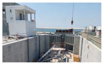
Engineering and fabrication for the project are now complete and the installation phase is underway. The four gates have been placed in position and the next phase will include the installation of walkways, floating pontoons, a hydraulic system to actuate the gates (HPU, tanks, cylinders and tubing, emergency HPU) and the fully-automated boat lock control system. Testing and commissioning will take place during Q3.
