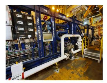
The piping component involved the development of six new MPD lines - as well as the reuse of existing lines - and the addition of Coriolis loops on the mud charging pumps. Pressure testing was carried out for all high pressure (HP) lines following the installation. Permanent lifting arrangements were also developed by 3C Metal to cater for assembly and removal of the MPD package onboard.
