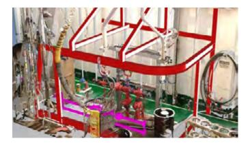
site installation of the supporting structure. Laser scans were completed while the drillship was in Pascagoula, Mississippi. The scans aided the engineering of all structural requirements and enabled all of the material and structures to be prefabricated. The successful installation resulted in a safer working environment for personnel onboard the drillship.
