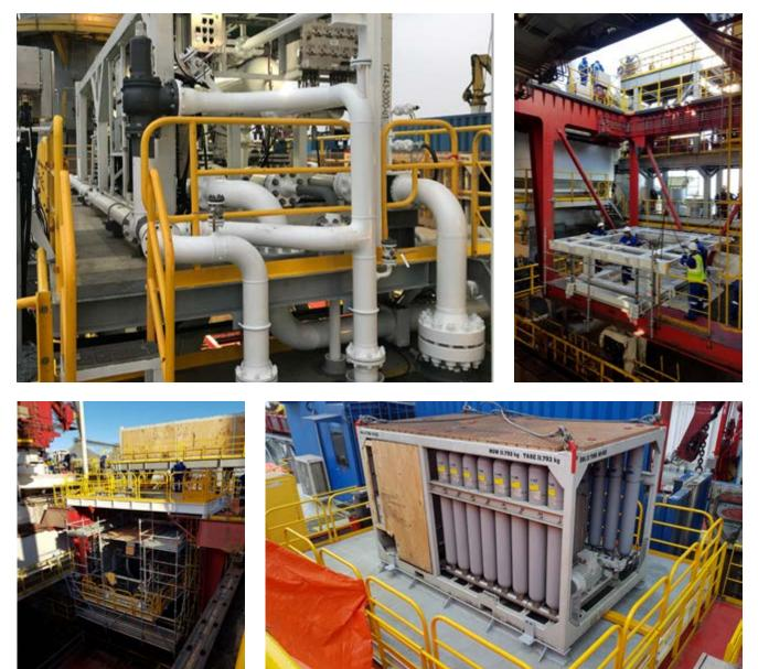
The work included a structure for the umbilical reeler, bridges to hold the hydraulic power units (HPU), three hose supports in a very tight moonpool, along with a deck extension and stiffening of the structures to house the large 35 ton AFGlobal MPD manifolds.
