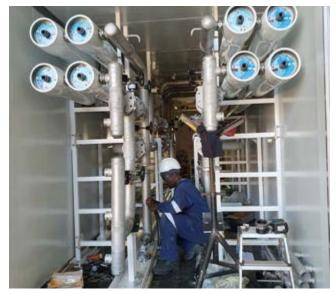
housings, UF modules, complete with the related piping, valves, instrumentation, pumps and other vessels installed in the 40ft shipping container.
