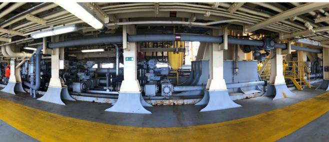
3C Metal carried out the initial laser scanning survey, the engineering, fabrication and installation. The scope of work included the modification of MPD piping (ICP spools flow lines), fabrication of spools and structural components, the installation of the new HPU and the supply and installation of support and cable trays.
