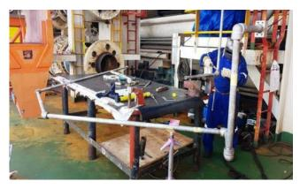
3C Metal supplied all the stainless steel 6,000 psi rated piping and fittings and fabricated all the different function routes onsite. All lines were made with dual seal hydraulic flanges, all tested to 9,000 psi and flushed down to NAS 6.
