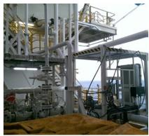
The scope of work included the engineering design, ABS class approval, prefabrication and installation required for the full system integration onboard the rig. In the initial stages of the project, 3C Metal deployed a team to carry out the onsite 3D laser scanning survey in Las Palmas. This aided the 3D modelling and accurate design for the structural integration and pipes routing.
