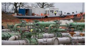
3C Metal were involved in the construction of counting and filtration installation; gas regulation; the construction of more than 1000m of pipeline ranging from 24 inches to 36 inches in diameter; and connections to six existing compressors.
