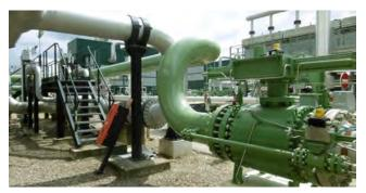
on behalf of Terega. These connections required 59 welds for pipeline ranging from 2 inches to 36 inches in diameter.
