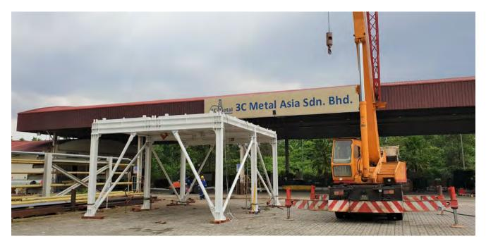
3C Metal demonstrated its full range of capabilities to complete the project by the required deadline. A laser survey allowed 3C Metal to accurately model the entire piping runs, thereby increasing prefabrication and reducing the installation time – this was a major challenge to conduct simultaneously with drilling operations.
