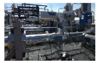
The salt system on a CSP plant utilizes Molten salts for thermal energy storage (TES). The ionic solids become liquids at elevated temperatures, offering exceptional heat transfer, chemical stability, and TES capability.
