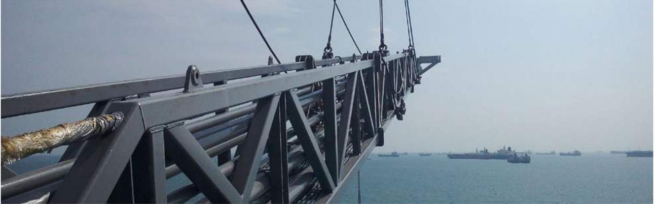
The burner boom structures were developed for a semisubmersible rig. The client commissioned 3C Metal Asia to provide the engineering, supply and fabrication of the two structures, the associated piping and all the necessary elements to connect it and integrate it onboard.
