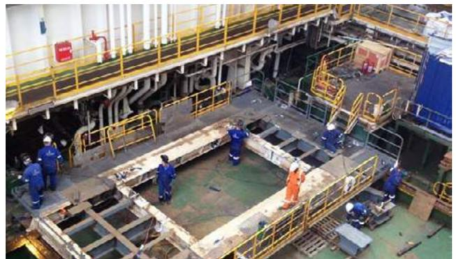
Seadrill requested the engineering, fabrication and installation of the IWOCS package. The main components of the project included pad eyes in the moonpool and DNV witness load tests; a platform for the GE deployment winch on the port side Xmas Tree stand; a modified platform in the center of the moonpool to land the IWOCS winch; modifications of the existing lines (LP and HP) to accommodate the IWOCS structure; and full electrical installation.
