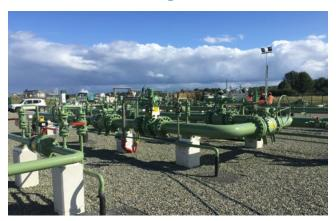
The RZL project involved diverting the main gas interconnections, operated by TIGF, from the former gas factory in the area. 3C Metal undertook the construction of four gas interconnection sites, including process equipment installation, such as gas counting, safety valves and coalescent filters. The work also involved the construction of six main pipelines, four horizontal drilling operations of 40m long, two horizontal directional drilling operations for cathodic protection.
