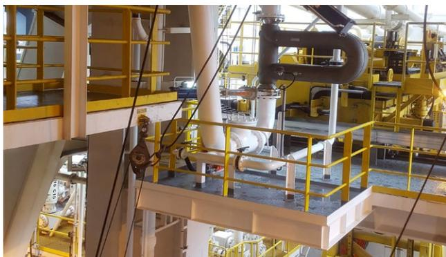
3C Metal was requested to follow the same integration route, where the Coriolis loop runs as a bypass of the rig's main flowline and is located beneath the drill floor near the diverter. 3C Metal provided a system on which all knife valves are pneumatically actuated and controlled by a pneumatic panel located on the drill floor. The panel contains an interlock that prevents the bypass valve from being closed when the valves on the loop are shut - mitigating the possibility of accidentally
